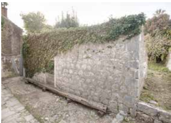
Spremište nasuprot mlinice
